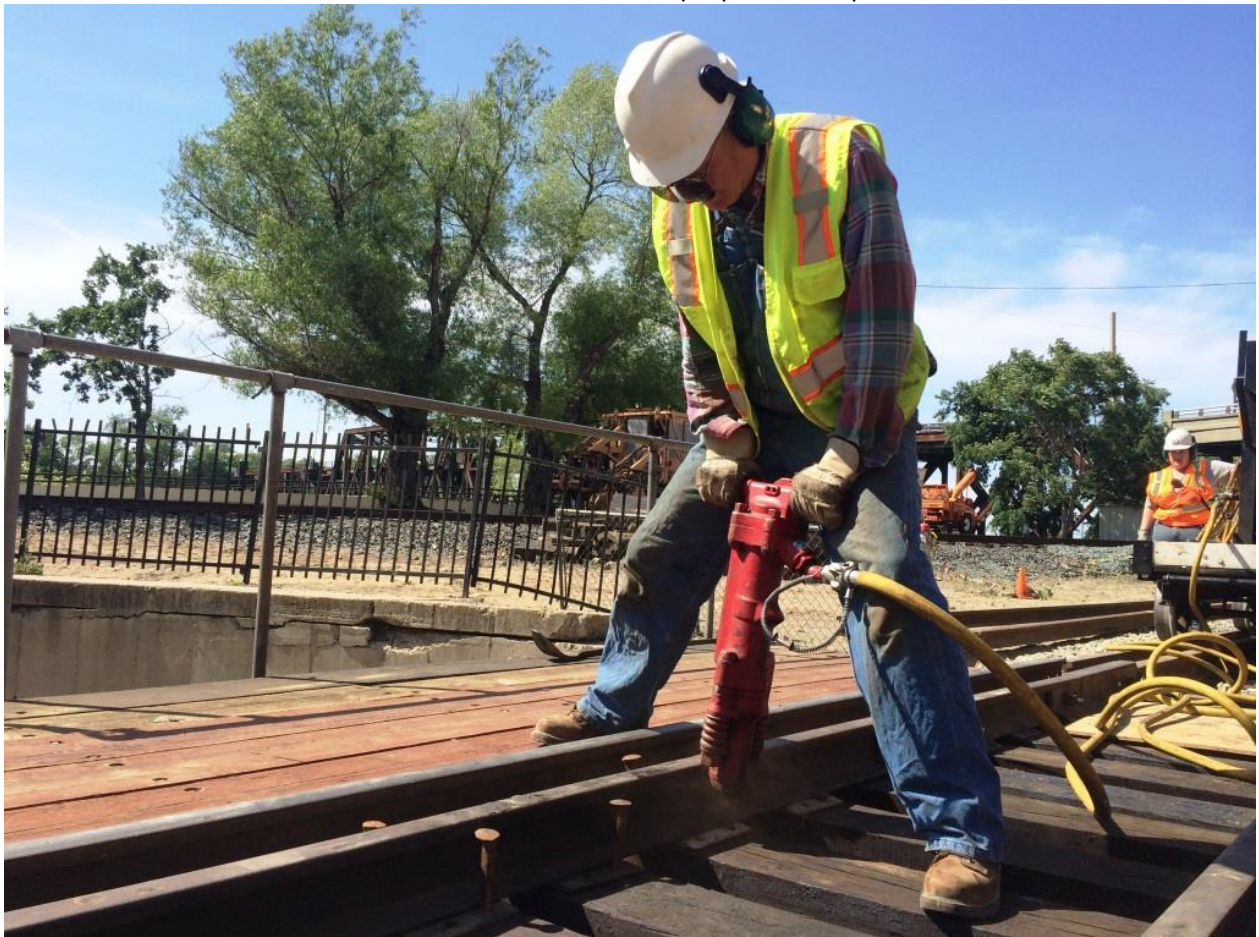
Steve spikes the narrow-gauge on the turntable with the pneumatic spiker
