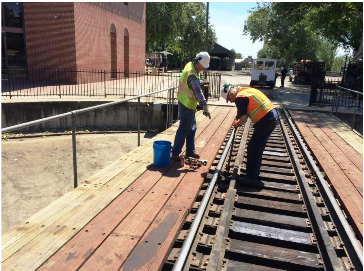
Steve provides appropriate bolt-tightening direction to Fred
