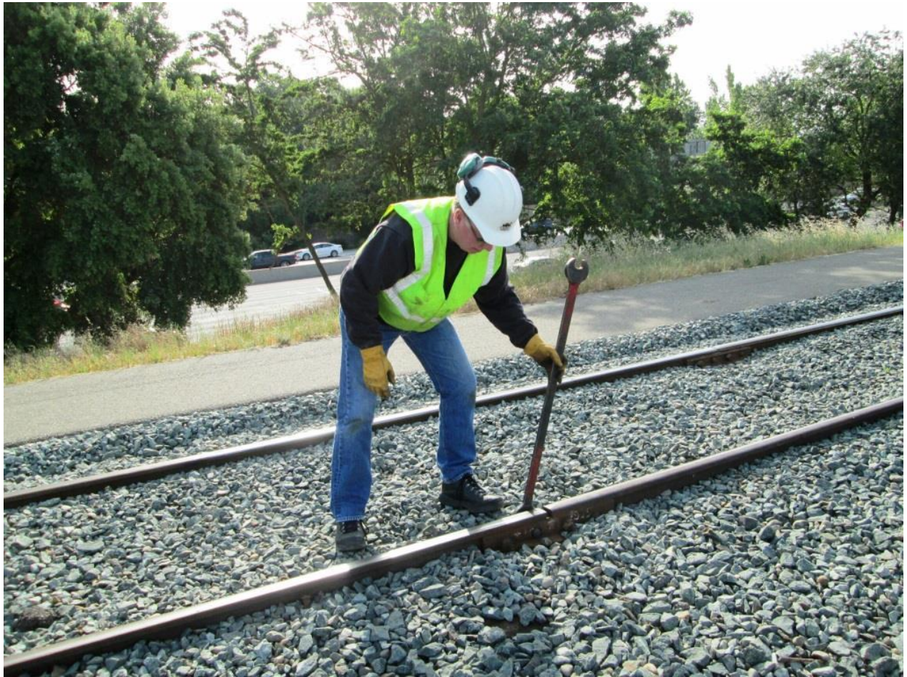
Ed replaces the broken bolt at Mile Post 2.5
